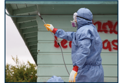
Lead-based paint remediation
